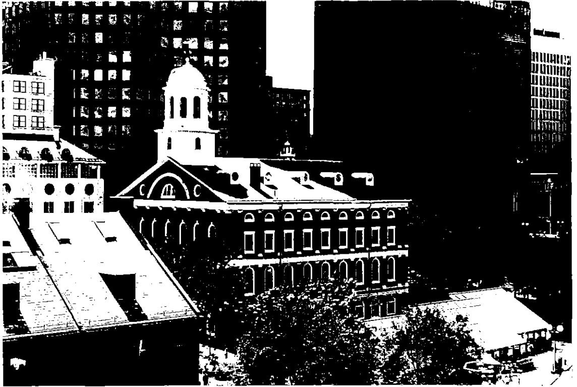
Faneuil Hall East and North Elevation August, 1994
