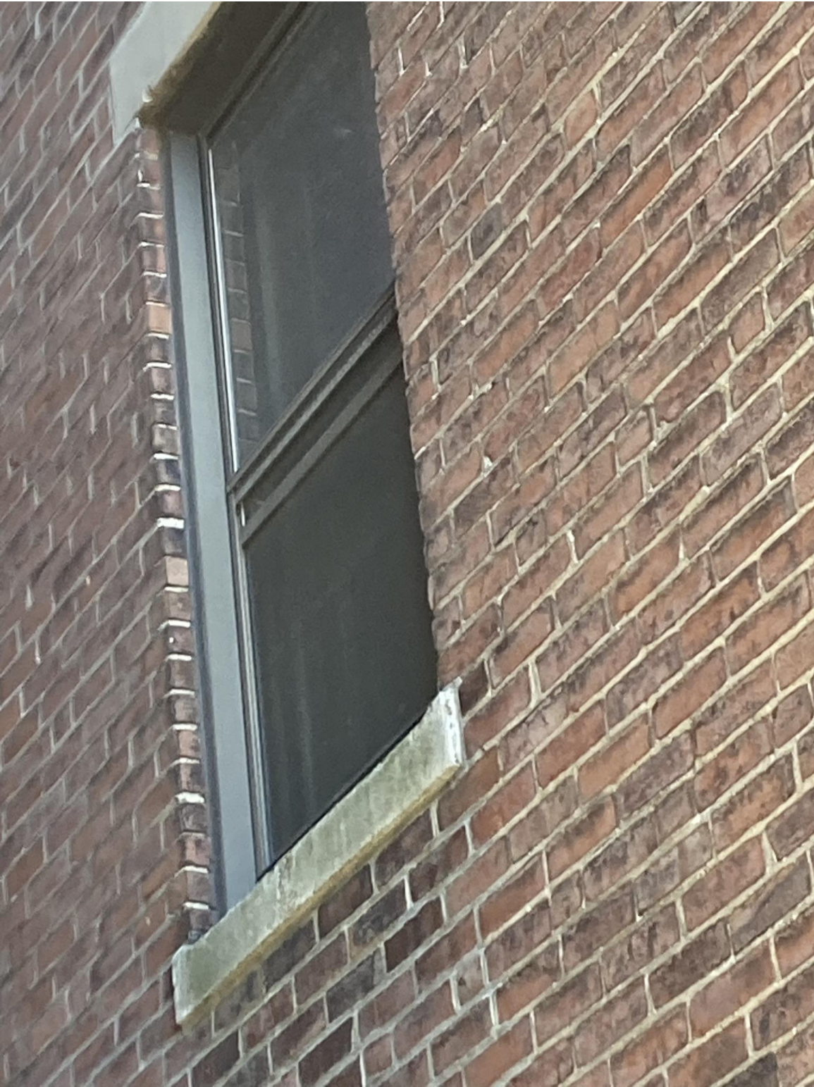
PREVIOUSLY REPLACED WINDOW
